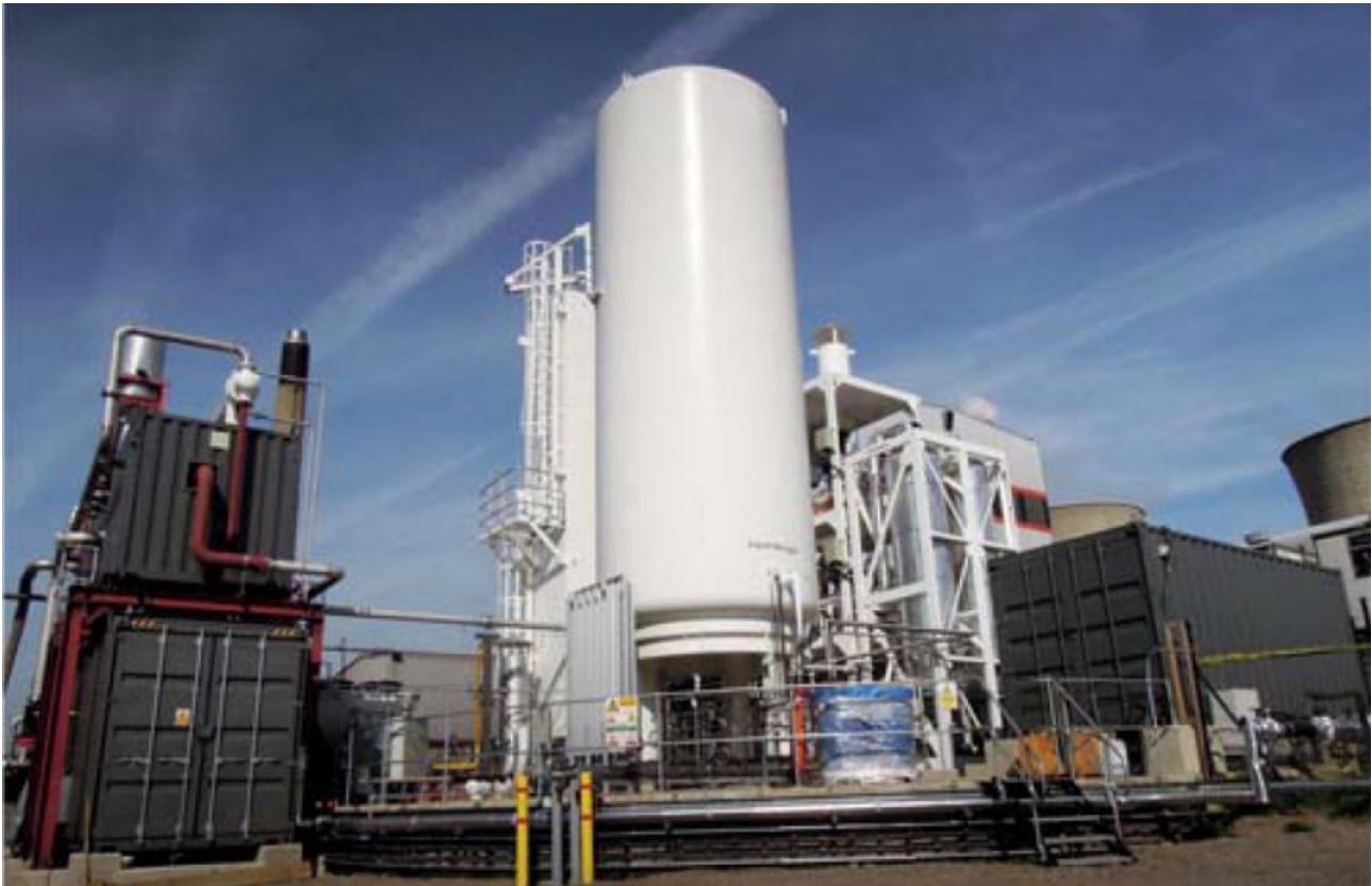
Figure i: LAES Pilot plant 350kW/2.5MWh
