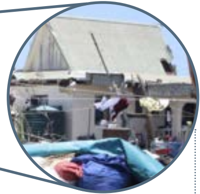
House destroyed by Cyclone Winston in Fiji in 2016. Note the relatively resilient concrete building in the background which was used for refuge during the disaster.
