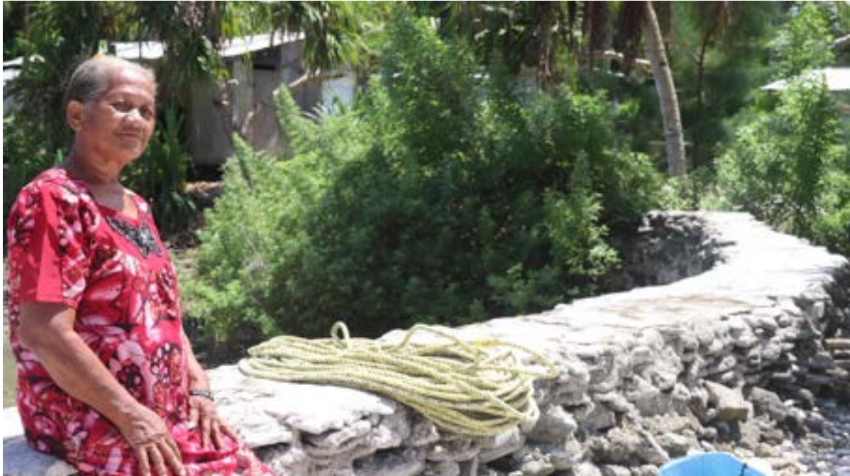
Seawall constructed with coral on Arno Island, Republic of the Marshall Islands.
