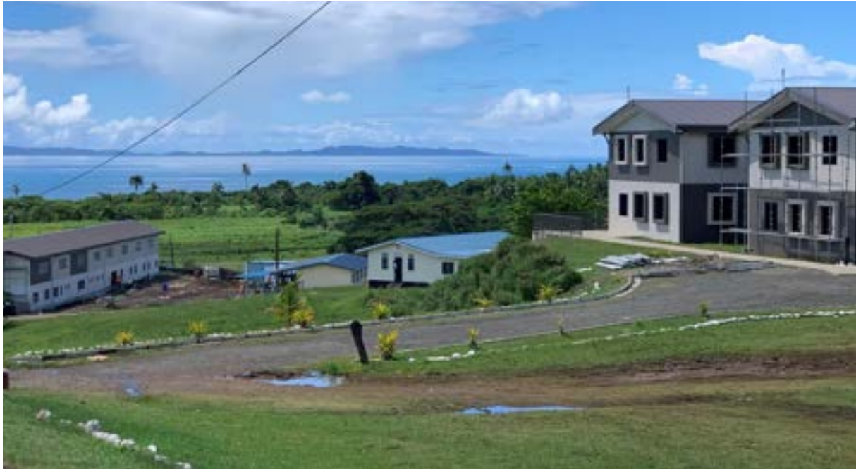
Reconstruction of a school in Fiji with resilient concrete materials designed to withstand future cyclones. Note: this photo was taken in 2023, seven years after the school was damaged by Cyclone Winston in 2016.
